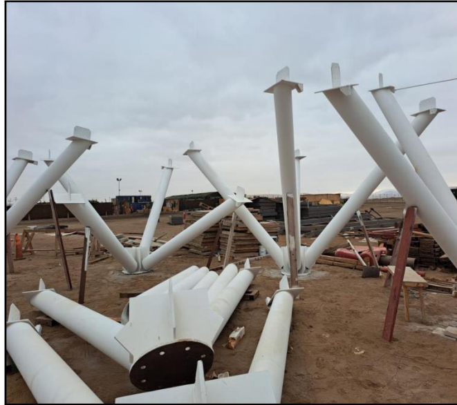
Foto-1: Vista General – Control Intumescente (DFT) Trepapodos
